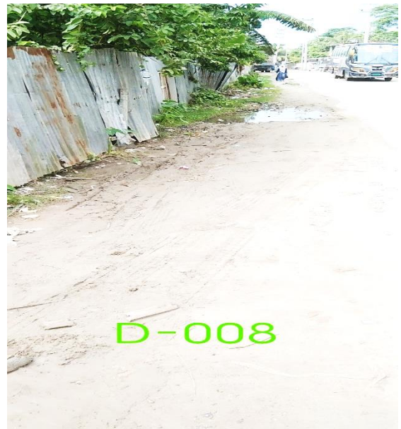
Photo , Haziganj- Drain -8
