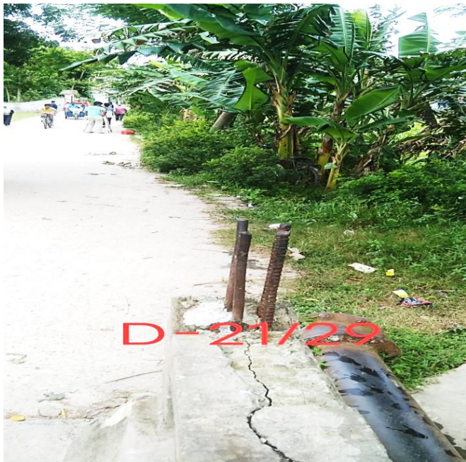
Photo , Haziganj- Drain -21
