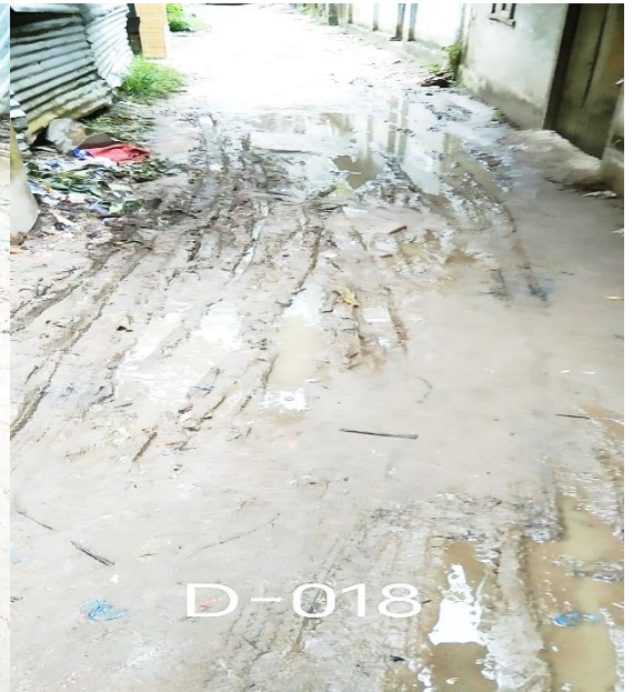
Photo , Haziganj- Drain -18
