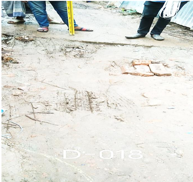
Photo , Haziganj- Drain -18
